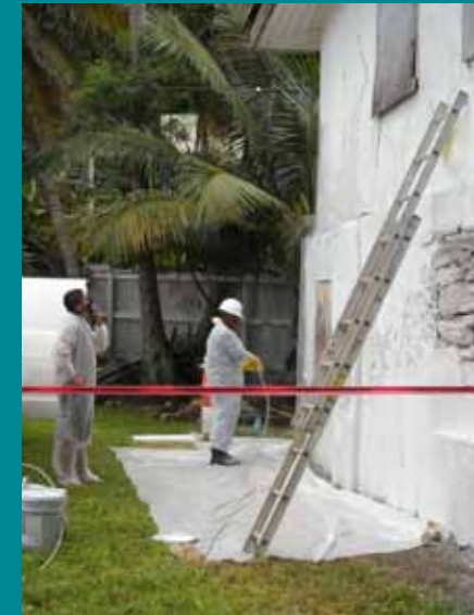
Lead based paint removal during demolition
