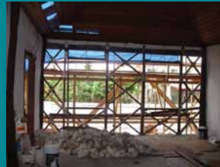
Deconstructing east wall. Note original stones to be reused.
