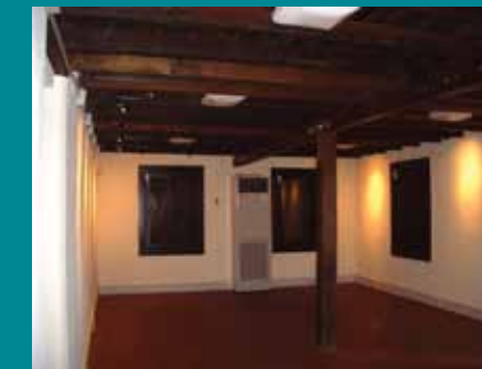
Completed lower floor showing new and original floor beams and salvaged 1982 floor tiles
