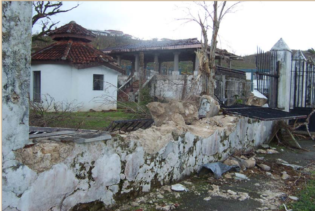
Mamposteria Fence walls at the Plaza de España (Guam and National Register site) were damaged during super typhoon Pongsona in December 2002. The roof of the Azotea (seen in the background) was also severely damaged by typhoon winds.
